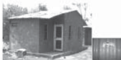
Fig. 5. Sisal fibre reinforced corrugated Roofing Sheets
